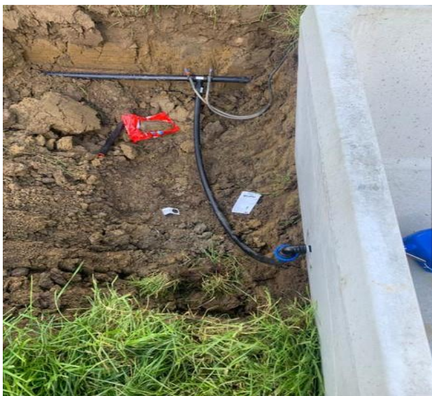
Connecting water pipes to trough
