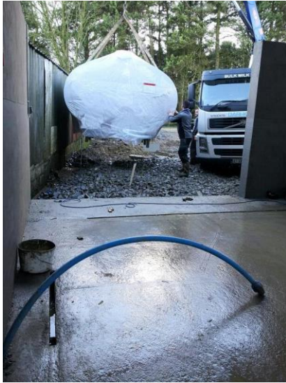
Installation of bulk milk tank prior to roofing of dairy
