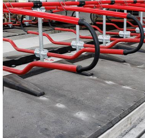
Cubicle mats installed
