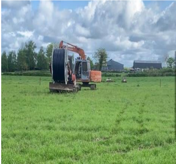
Installing water pipes on farm
