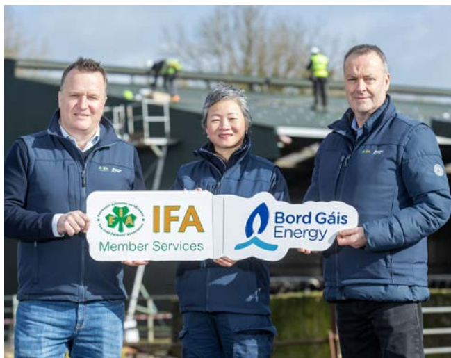
Pictured at the solar installation on the farm of Andrew McHugh, Co Longford is John Cussen, Bord Gáis Energy, Christina Ngo, Bord Gáis Energy and Peter Clarke, IFA.
